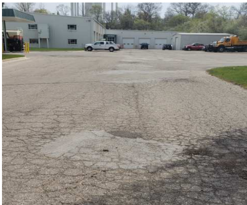
Public Works Site
