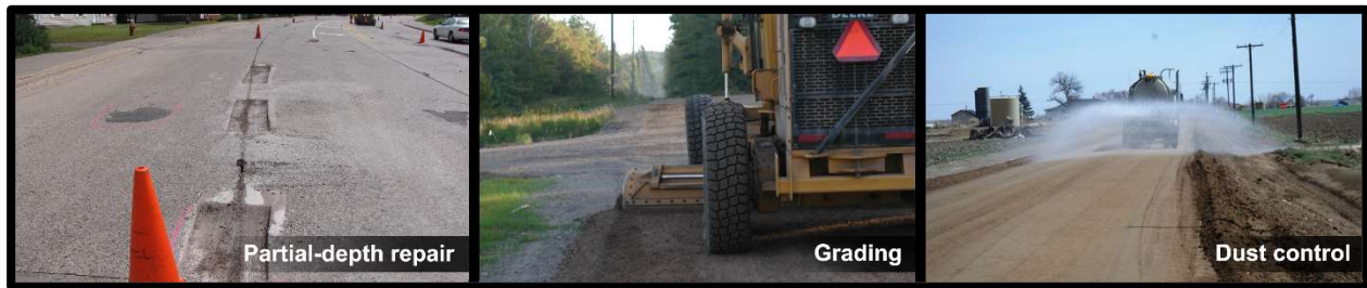
Figure 5: Examples of capital preventive maintenance treatments, cont'd—(from left) concrete road prepared for partial-depth repair, gravel road undergoing maintenance grading, and gravel road receiving dust control application (dust control photo courtesy of Weld County, Colora, weldgov.com).
