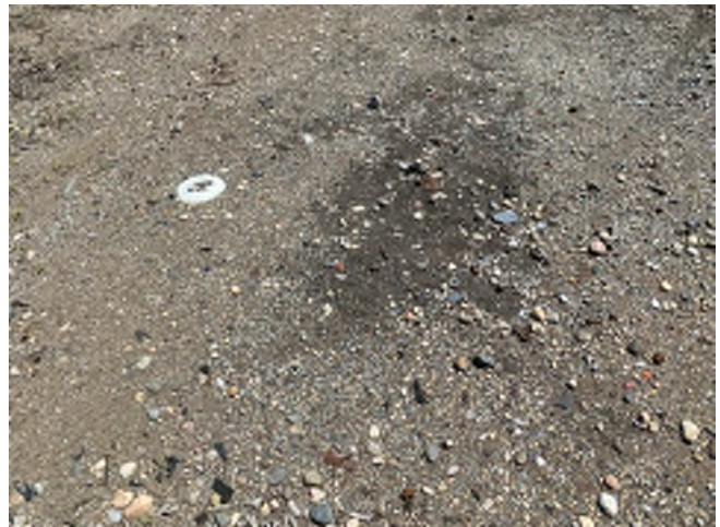
Petroleum stained soils
