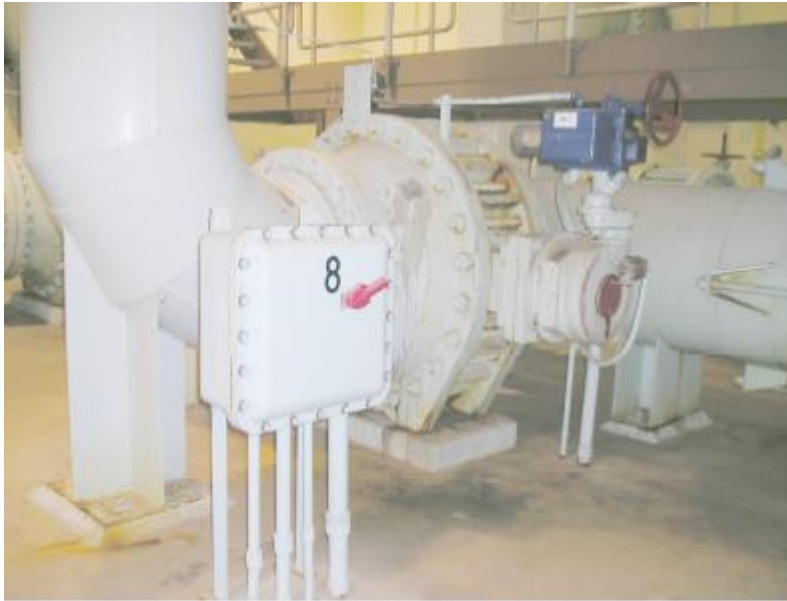
HIGH SERVICE PUMP NO. 8 DISCHARGE VALVE
