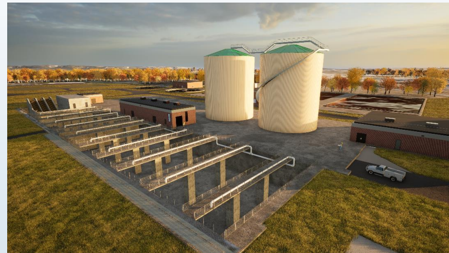
Alternative 1: Steep Cone Cylinder Anaerobic Digester Concept
