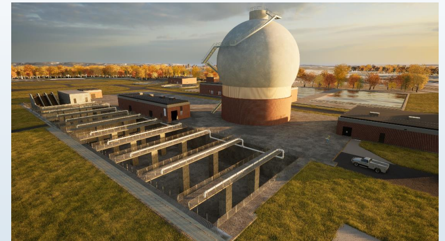
Alternative 2: Egg-Shaped Anaerobic Digester Concept
