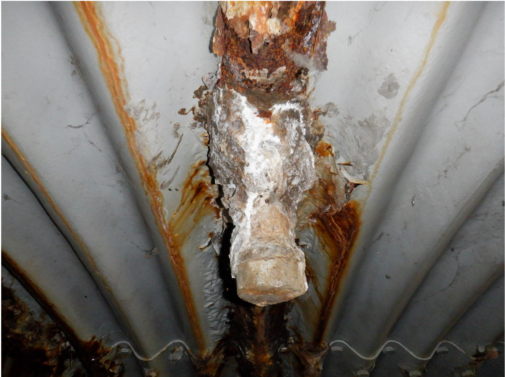
PREVIOUS HOLE IN WEST WALL OF EAST BARREL FILLED WITH HYDRAULIC CEMENT
