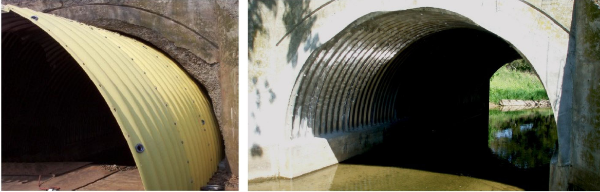
Example culvert lining project
