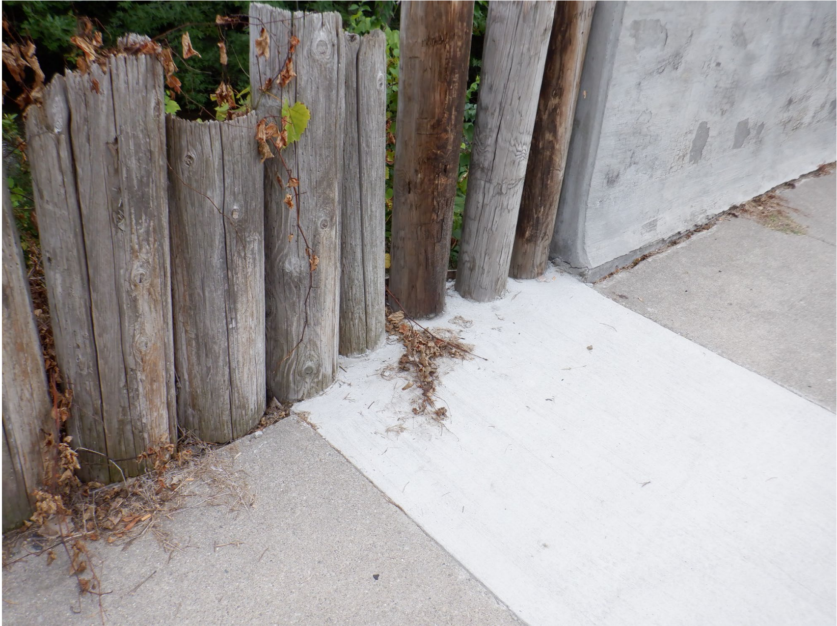
NEW SIDEWALK SECTION IN SOUTHEAST QUAD
