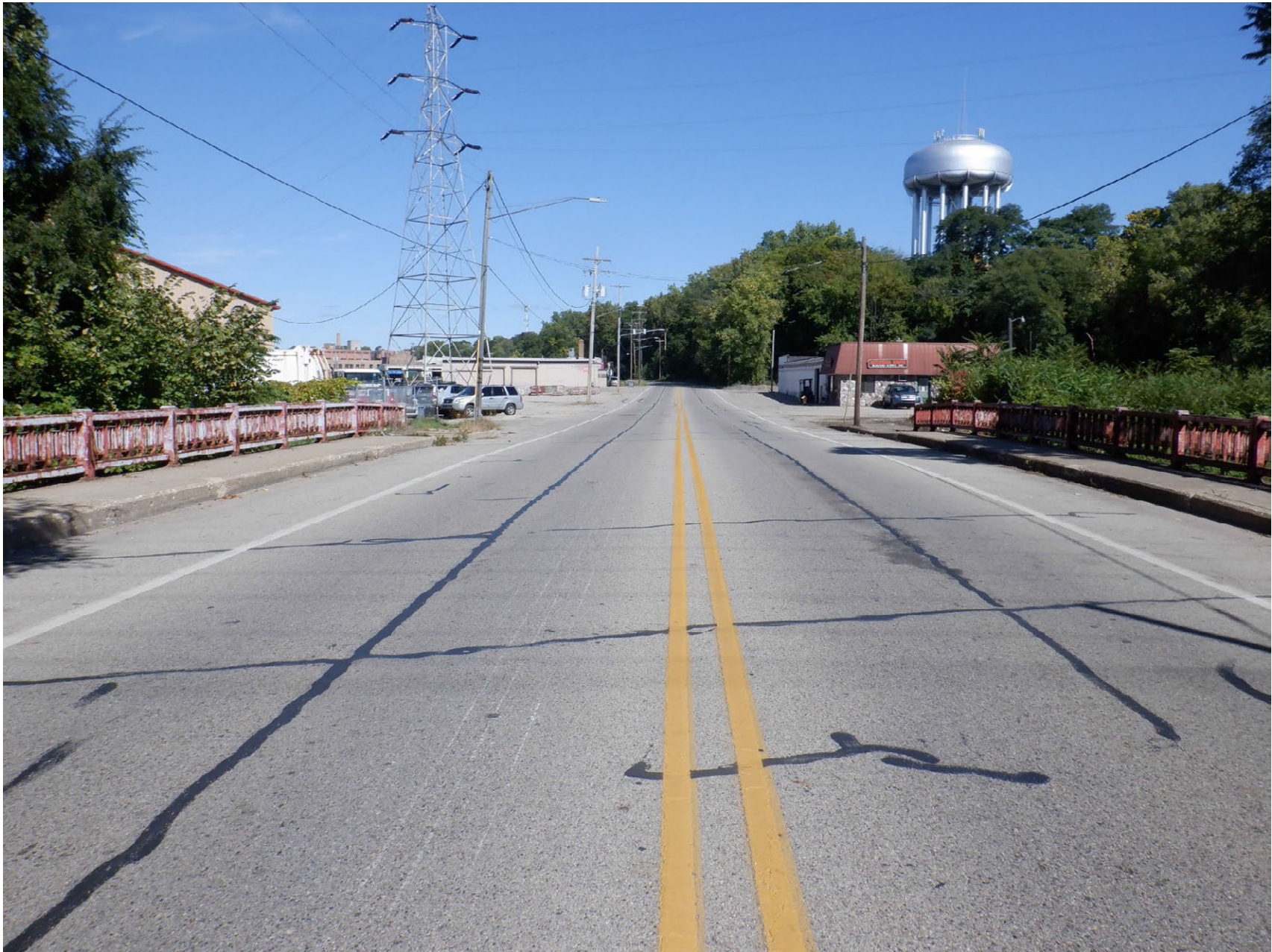
BRIDGE SECTION LOOKING NORTH
