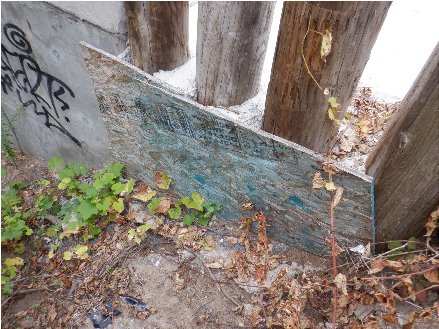
PLYWOOD BOARD HOLDING FILL IN SOUTHEAST QUAD
