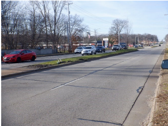
Road section over culvert
