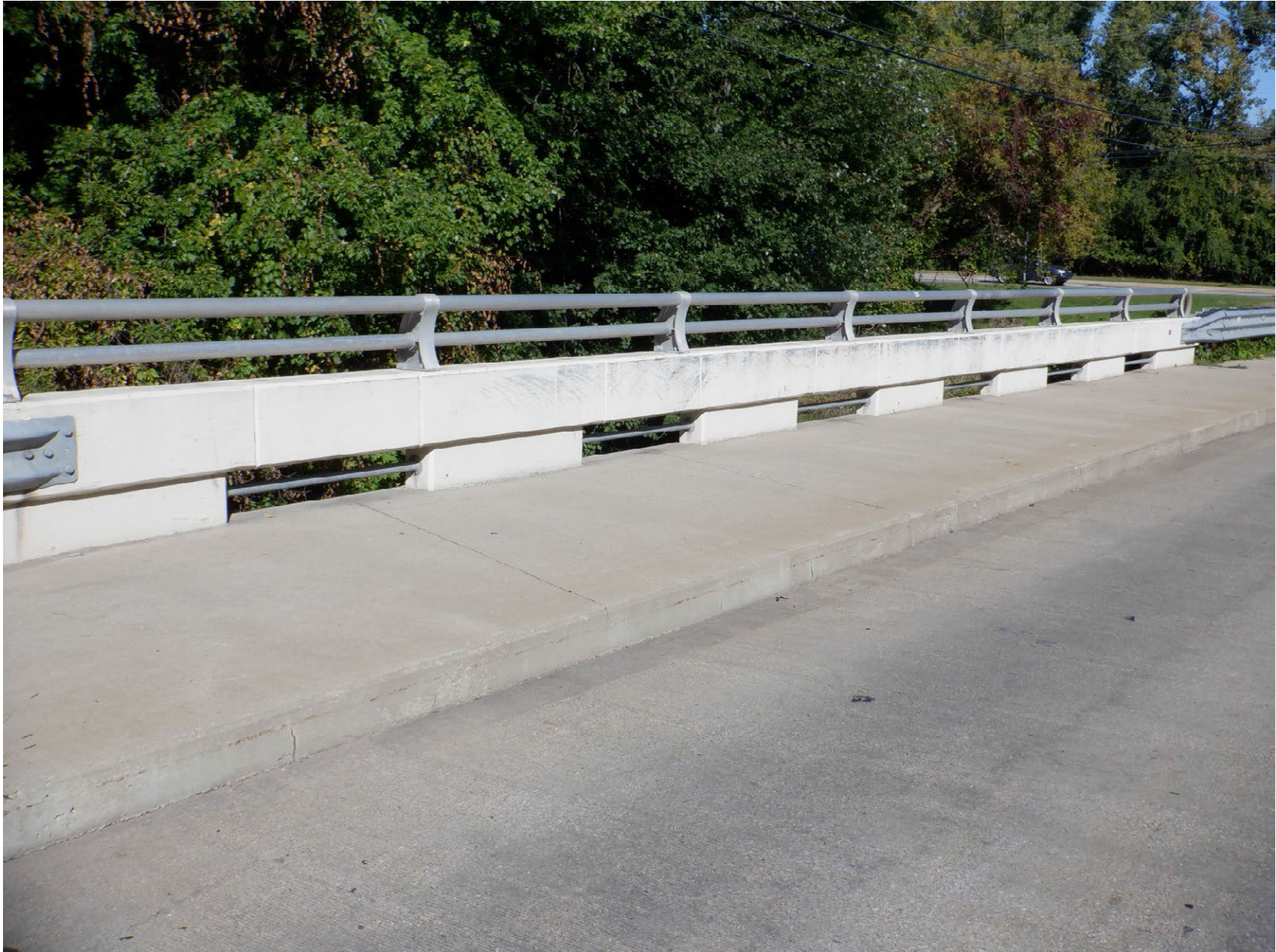
BRIDGE RAIL AND SIDEWALK ELEVATION
