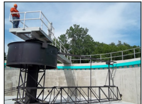
One of Several New Final Clarifiers &
