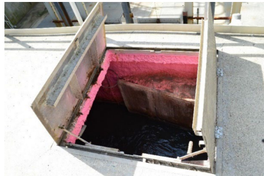
Newly Repaired – Coated Channels
