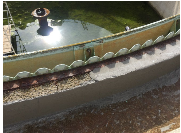
Concrete Trough Repairs in Progress
