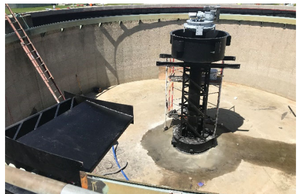
Replaced Final #3 Mechanism & Internals
