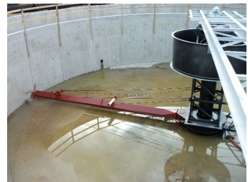
Installation of Final Tank Mechanism
