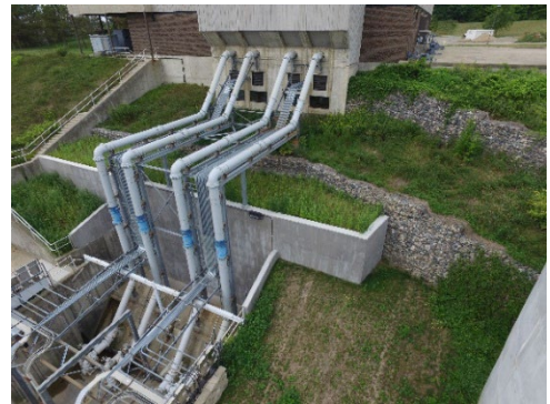
New Concrete Wall Aerial View
