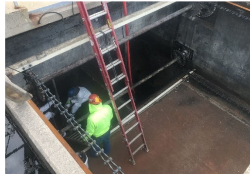
Primary Mechanism Replacement
