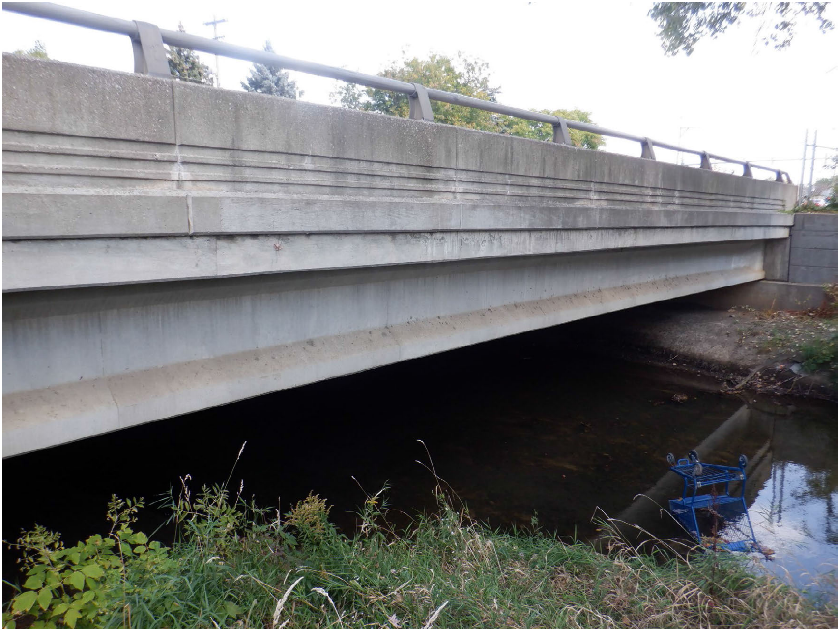
SOUTH BRIDGE ELEVATION
