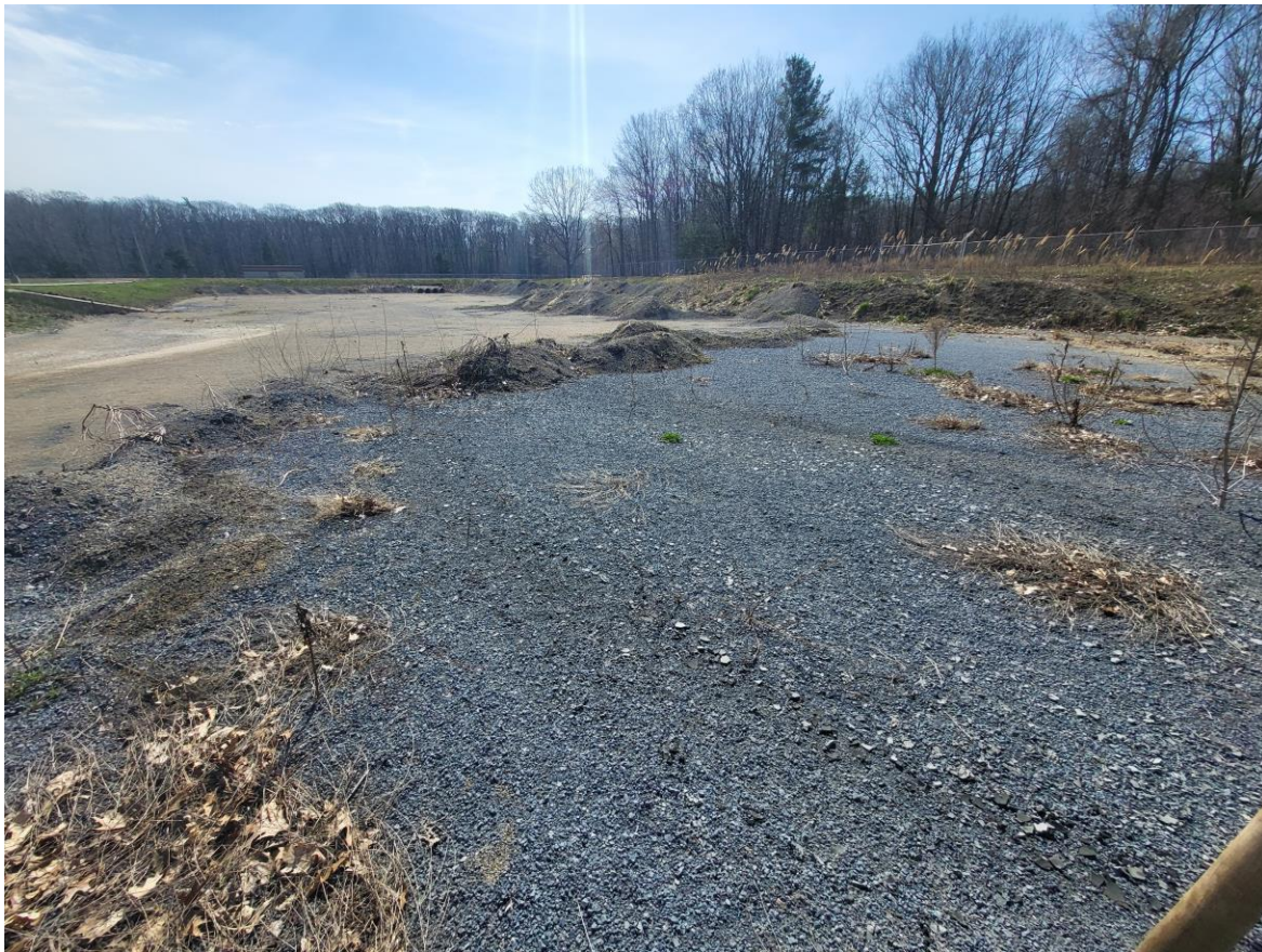
South Drying Bed at the Drinking Water Plant
