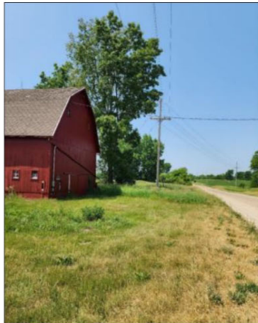
Approved overhead permanent service and clear path.
