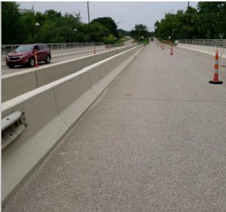
TYPICAL BRIDGE AFTER EPOXY OVERLAY
