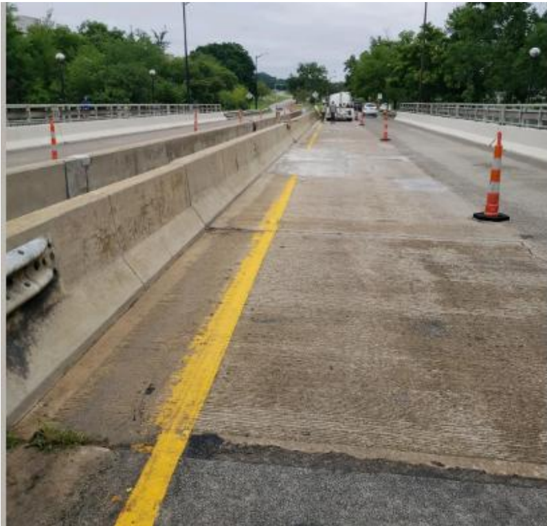
TYPICAL BRIDGE BEFORE EPOXY OVERLAY
