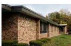
GAINES TOWNSHIP BRANCH 421 68th St. SE Grand Rapids, MI 49548
