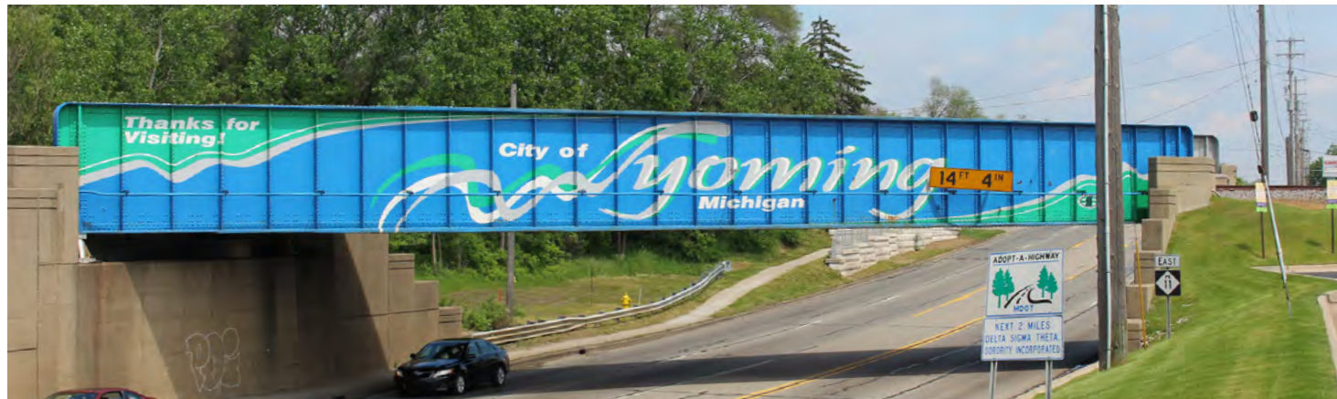
Example of Entry Point Enhancement in Wyoming, MI
